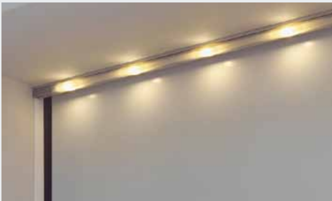
LED light strip fitted on the lintel
